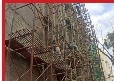
BLOCK J – External plastering in progress
