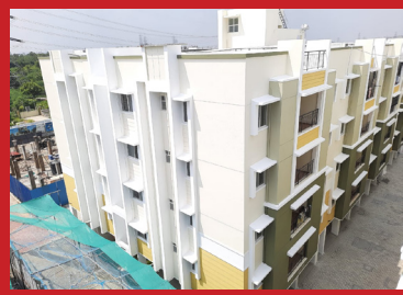
BLOCK B – Completed View
