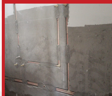
BLOCK J – Third Floor Toilet plumbing in progress
