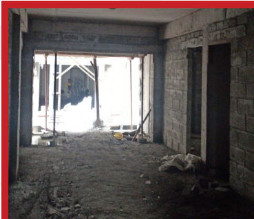
BLOCK K – 1st Floor Block Work
