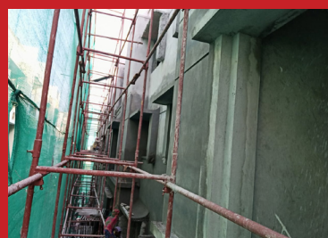
BLOCK J - External plastering in progress
