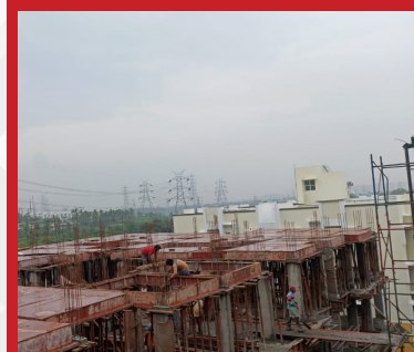
BLOCK K – Terrace Floor Slab shuttering work in progress
