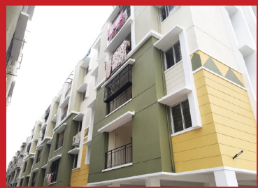
BLOCK C – Completed View
