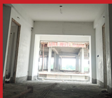
BLOCK J - Third Floor Putty work in progress
