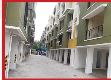
BLOCK C – Completed View
