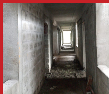
BLOCK K – 1st Floor Block Work
