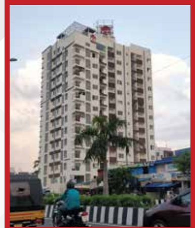
Completed View From OMR
