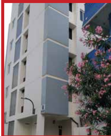
BLOCK B - Front View
